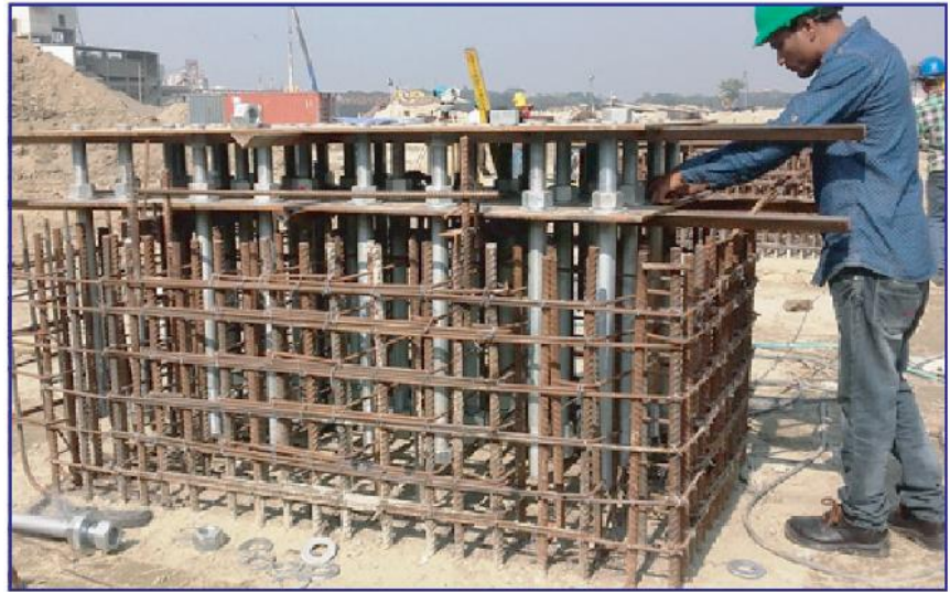
Anchor Bolt Setting
