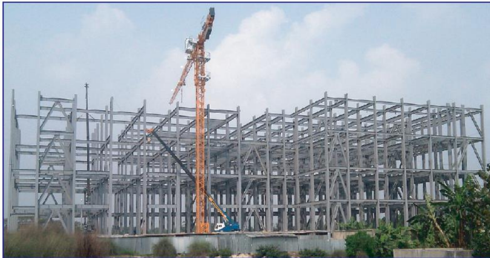
Erection with Tower Crane
